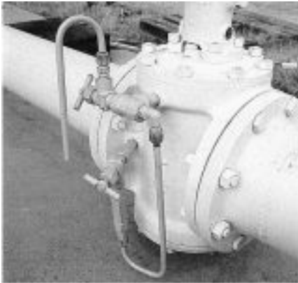
MANUAL BLEED WITH THERMAL RELIEF (MTR)
