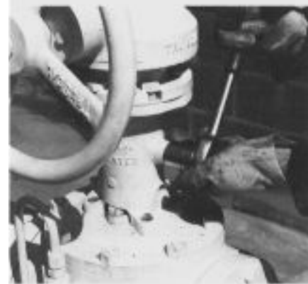
CAM PIN REMOVAL
