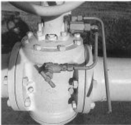
AUTOMATIC BLEED VALVE (ABV)
