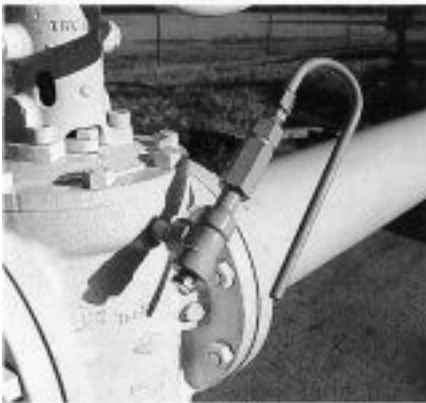
THERMAL RELIEF TO ATMOSPHERE (TRA)
