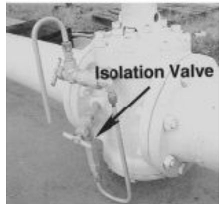
MANUAL BLEED WITH THERMAL RELIEF (MTR)
