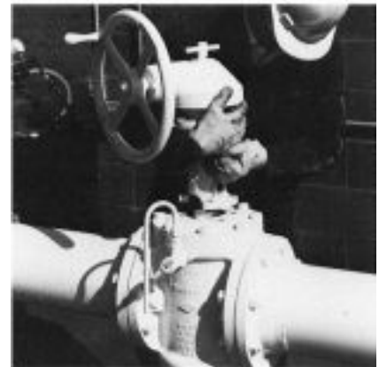
OPERATOR REMOVAL
