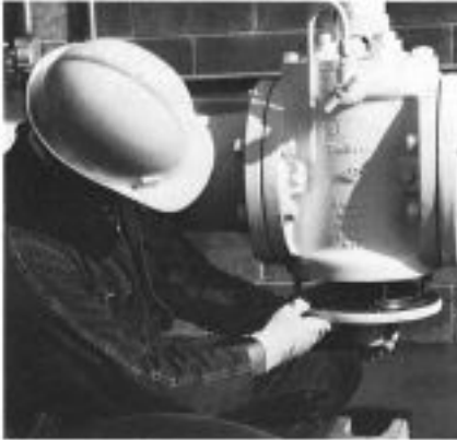
LOWER PLATE REMOVAL
