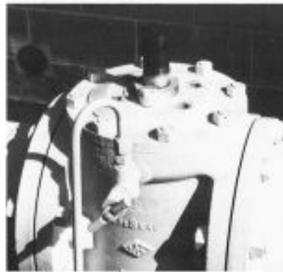
VALVE WITH OPERATOR REMOVED
