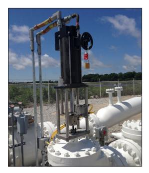
directly to a linear force. This unique design provides high force and fast response needed for the application, as well as long life to minimize maintenance. Controls for the actuator were provided by Rockwell Automation, seamlessly integrating the Exlar valve actuator into the overall pump station control. The control scheme also includes continuous diagnostic capabilities; providing information on the health of the valve as well as the actuator
